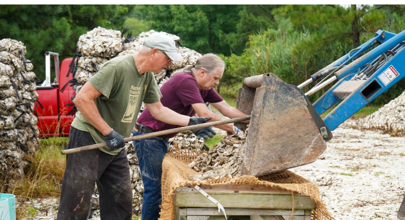
Volunteers finish creating a burrito of oyster shells to be used in oyster reef construction.
