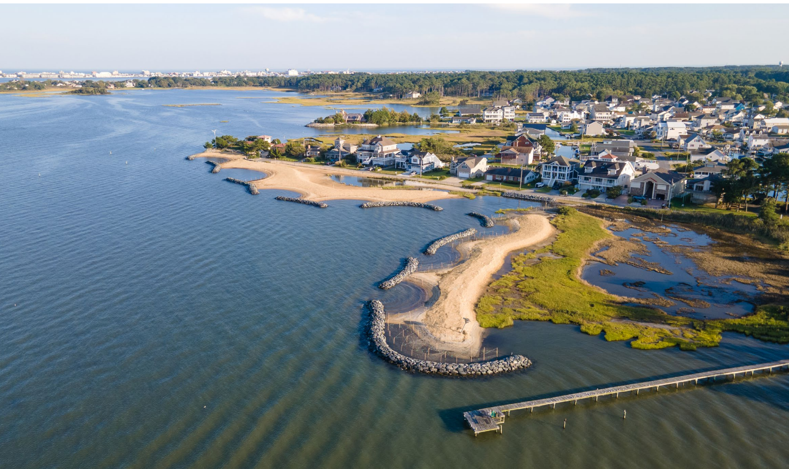
Aerial view of the Selsey Road Living Shoreline project on the Isle of Wight Bay in West Ocean City, Maryland.
