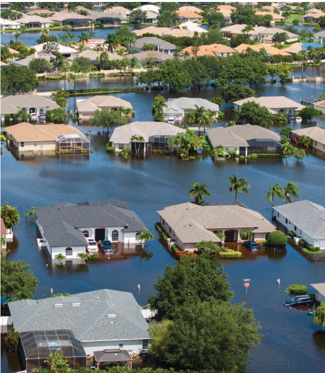
Flooded houses from Hurricane Debby rainfall water in Laurel Meadows community in Sarasota, Florida.
