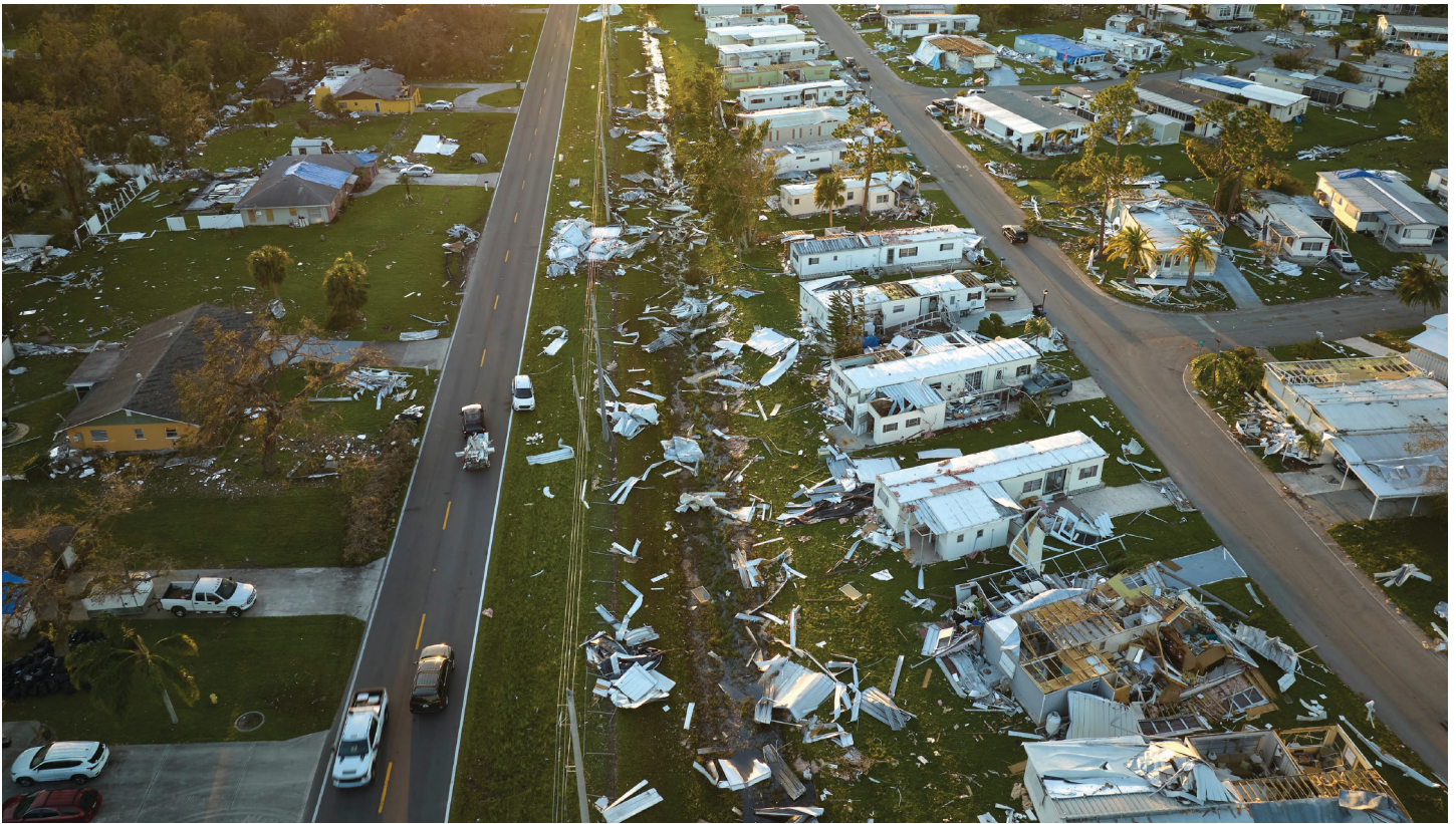
Severely damaged houses in a Florida mobile home residential area after Hurricane Ian. Credit: Shutterstock
