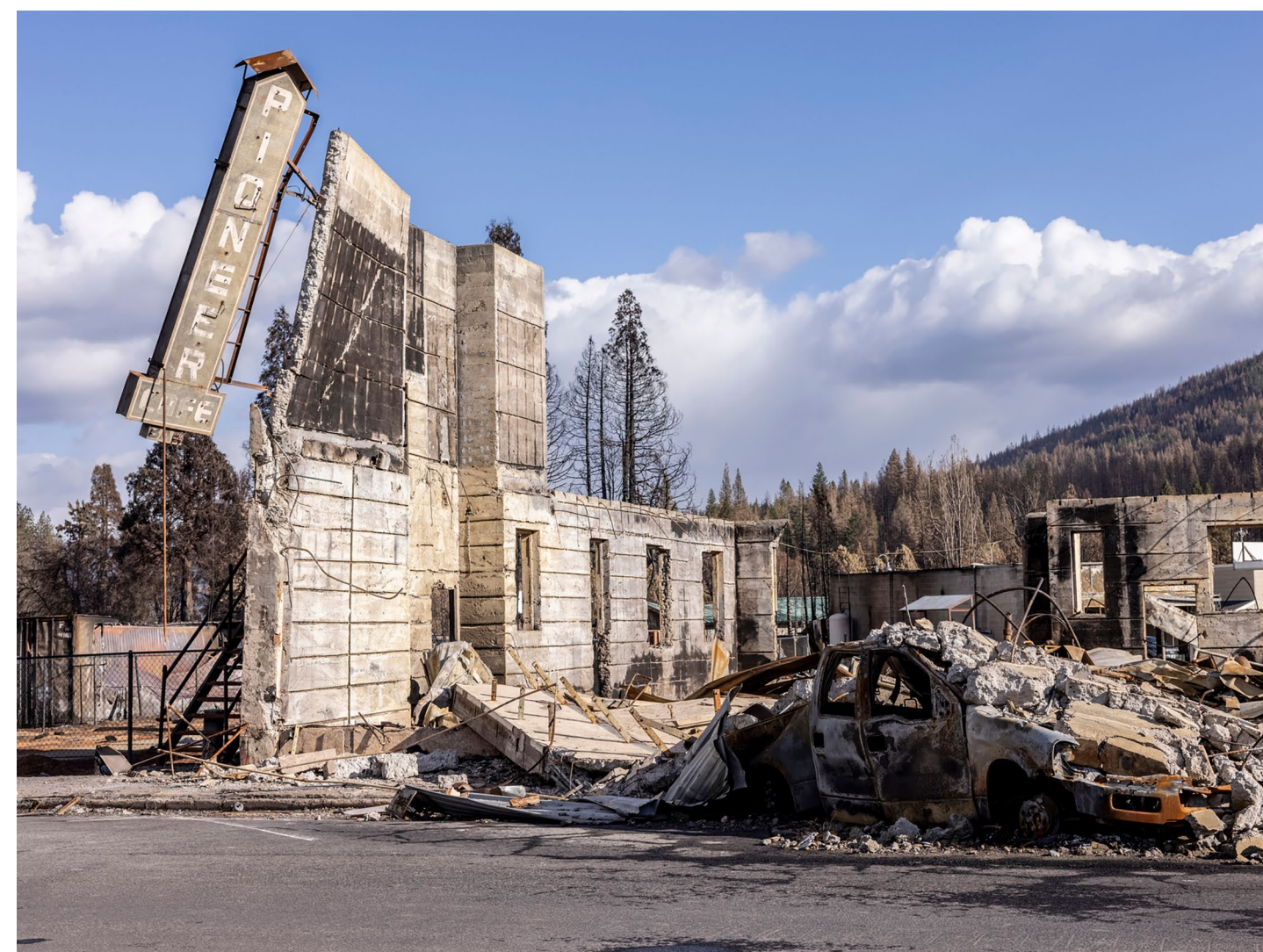
The Dixie Fire of 2021 destroyed most of Greenville, California. Credit: JasonDoiy/iStockphoto
